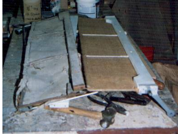
The new shutters under construction, and the one surviving original on which they are based
