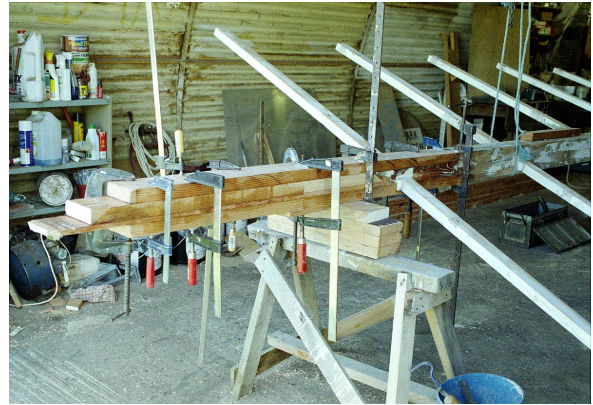
Lengthening the sail whip by laminating new material onto the heel
