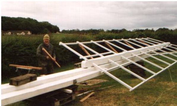
Assembling the new sails on the ground and fitting backstays
