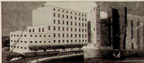
Ideally situated. The facilities at our disposal enable us to guarantee uniform quality and service.
