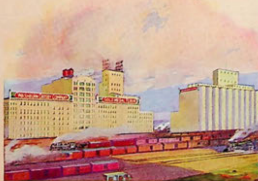
GOLD MEDAL MILL NUMBER ONE Minneapolis, Minnesota Another of the Gold Medal Mills operated at the principal sources of wheat supply.
