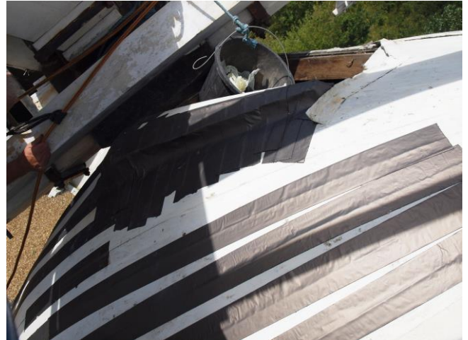
Fig.7 Covering large hole caused by roof distortion
