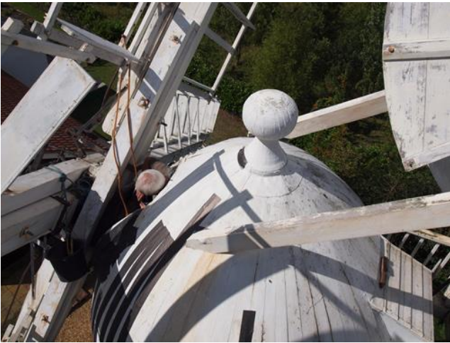
Fig.6 Covering gaps in the roof with flash band
