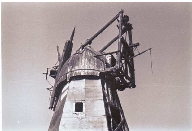
Fig.2 Under restoration, 1984 (b)
