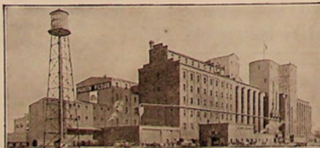
Winnipeg Plant (St. Boniface) Daily Capacity, 5,000 Bbls
