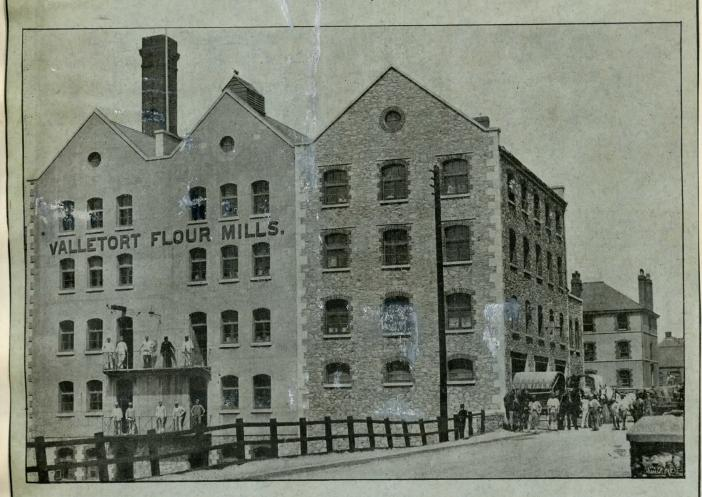
The above illustration shows the Plymouth Mills of Messrs. Hosken, Trevithick, Polkinhorn & Co., Lim. This Mill contains a Twelve Sack per Hour Roller Plant on the Simon System and a complete Wheat Preparing Plant, consisting of the Simon Patent Wheat Washer and Stoner and Patent Wheat Dryers, &c.
