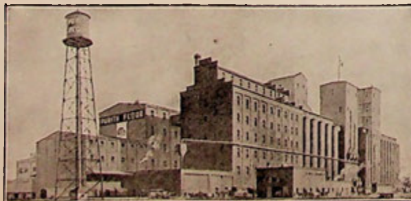
Winnipeg Plant (St. Boniface) Daily Capacity, 5,500 Bbls
