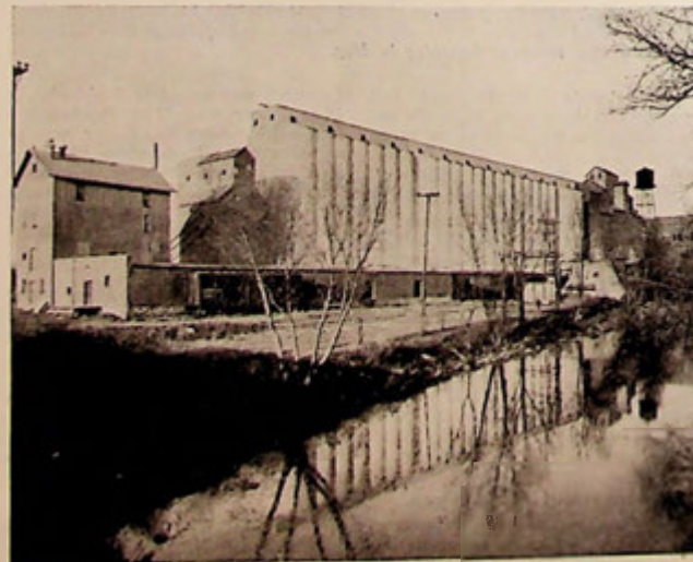
AN important addition to the country mill storage in the Northwest. This imposing battery of tanks, with a capacity of 1,500,000 bus, is part of the plant of the King Midas Mill Co., at Hastings, Minn., and was completed late last fall.
