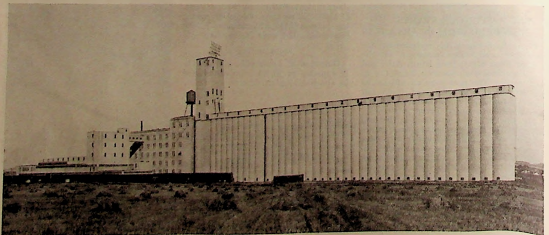
ENLARGED mill and wheat storage of the Robin Hood Mills, Ltd., at Saskatoon, Sask., was recently completed. The mill is in two units of 1,500 bbls each, with total storage capacity of 1,400,000 bus. The buildings and tanks are of concrete construction, and electric power is used throughout. Adjoining the mill is a warehouse, with floor space of approximately 31,000 square feet. The plant, one of the most modern in western Canada, presents a unique appearance, with its huge battery of storage tanks, and wheat field in the foreground.
