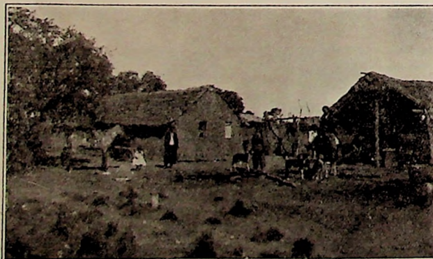
Typical Small Argentine Farm House and Buildings, Thatched Roof Here Taking the Place of the Usual Corrugated Iron
