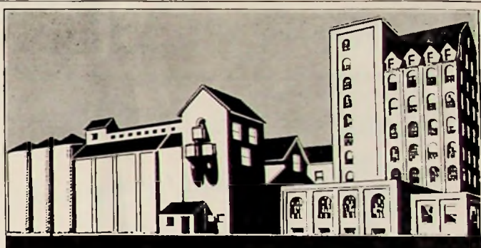
Half a Century of Milling Progress
