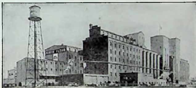
Winnipeg Plant (St. Boniface) Daily Capacity, 5,500 Bbls
