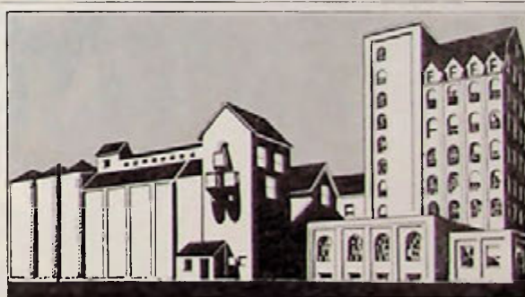
Half a Century of Milling Progress
