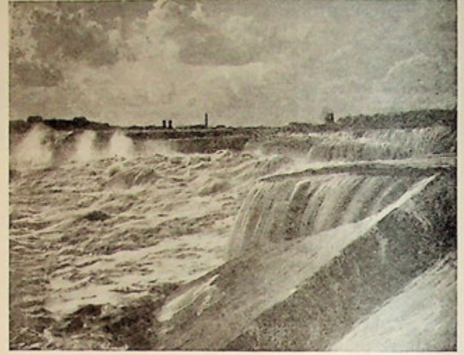
The Falls of St. Anthony, Prior to Their Final Harnessing, in 1871, to the Needs of the Minneapolis Flour Milling Industry
