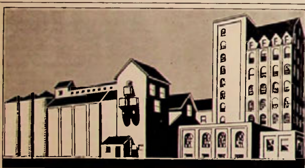
Half a Century of Milling Progress
