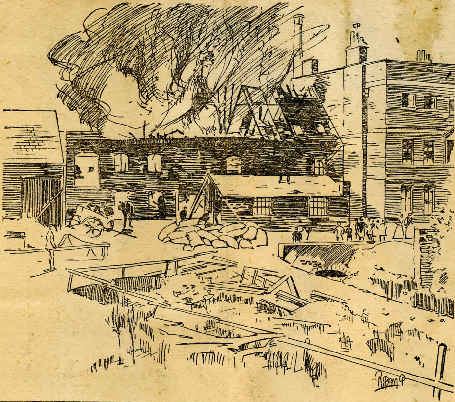
MILL FIRE IN THE ISLE OF WIGHT: REMOVING SACKS FROM THE BURNING BUILDING. (From a Photograph by Charles Knight, Newport, Isle of Wight.)
