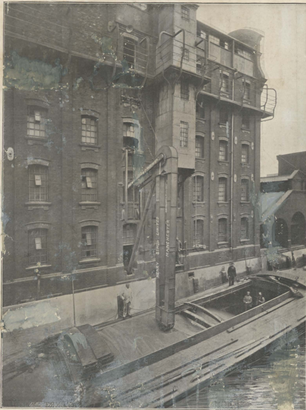
SHIP ELEVATOR AT THE MILLS OF MESSRS. MARRIAGE, NEAVE & Co., LTD., BATTERSEA.
